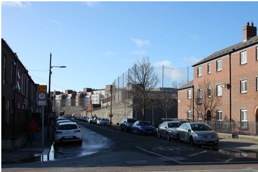
FIGURE 5-9 THE VIEW ALONG ORIEL STREET UPPER FROM THE NORTH
