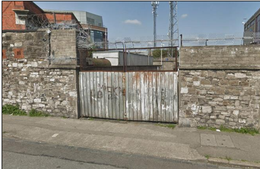
PLATE 13-3: BOUNDARY WALL ALONG ORIEL STREET WITH OPENING AND MODERN ADDITIONS, FACING NORTHWEST
